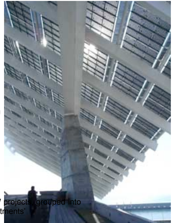
The forum in Barcelona with its photovoltaic sun shading system
