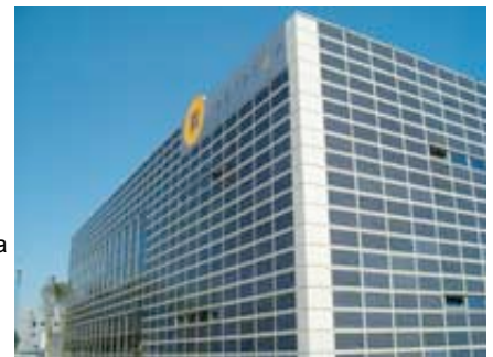
The PV-clad walls of a solar cell manufacturing plant in Malaga, Spain ISOFOTÓN
